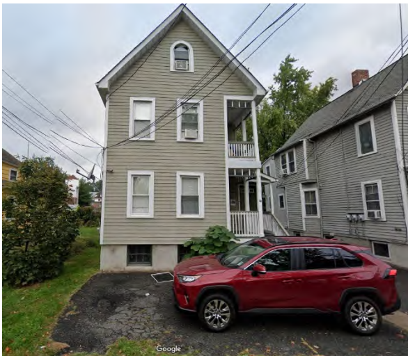
Figure 19: Three-family home at 14 Miller Street.
