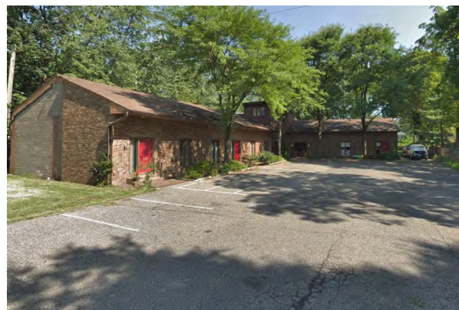
Figure 26: Office building on Beldin Place.
