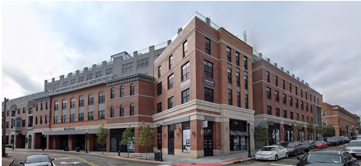
Figure 3: Two South Willow which contains twenty affordable rental units.
