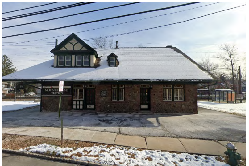
Figure 19: Mountain Avenue Train Station.
