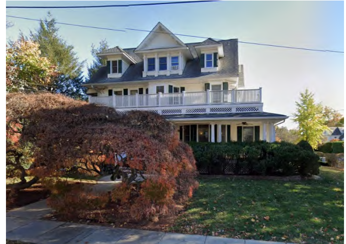
Figure 27: Little Nursing Home at 71 Christopher Street.
