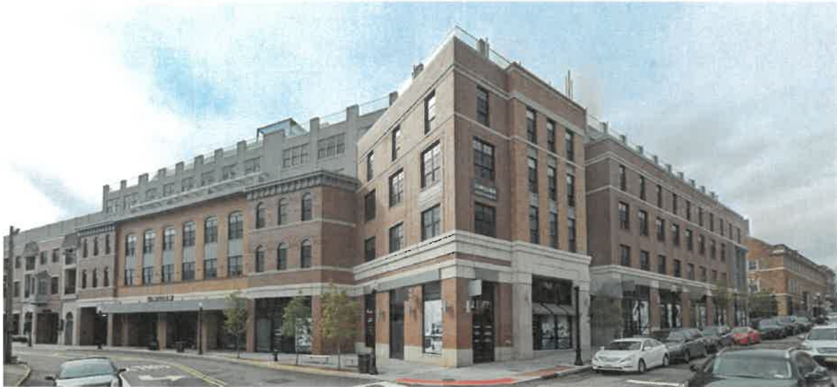
Figure 3: Two South Willow which contains twenty affordable rental units.
